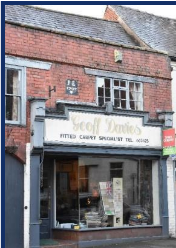
Figure 13 A townhouse on Willow Street dated 1707 with a late 19th-early 20th century shopfront inserted on the ground floor. Today we might opt for a design which doesn't obscure so much of the upper floors, but the large fascia and timber entablature is now part of the building's history.
