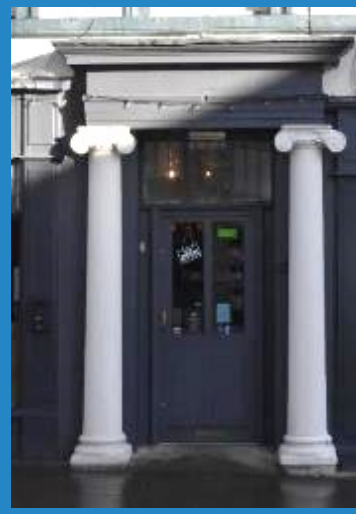
Figure 23 Entrance retains symmetry and classical features. Leg Street.
