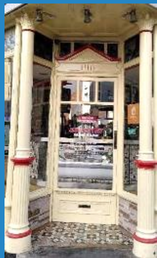
Figure 21 Well preserved entrance on Albion Hill.
