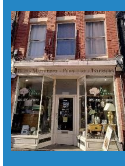
Figure 25 Mullions provide visual continuity with the upper storey windows to this property on Bailey Street.
