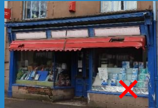
Figure 44 Here, a Dutch canopy has been installed instead of utilising the boxed blind which is still in place. Upper Church Street. Henry Thomas.
