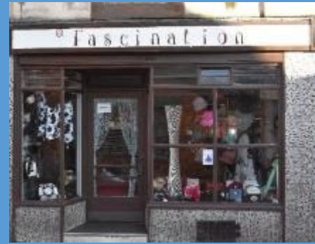
Figure 4 7-9 Leg Street contains a 1930s shopfront in a 'traditional style' but constructed in metal rather than timber.
