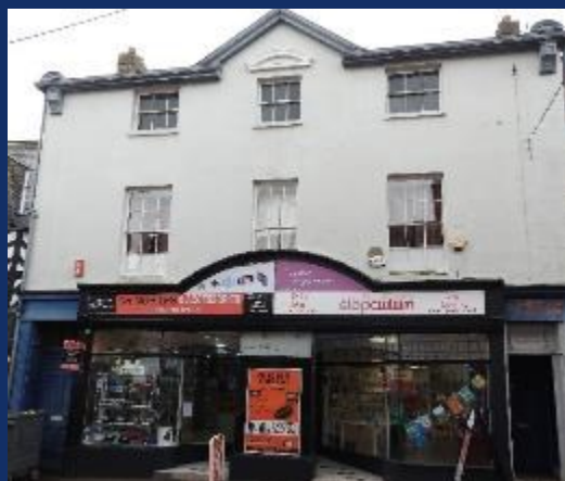
Figure 12 Today, the shopfront with its distinctive arched fascia board survives but the ground floor has been split into two shops. The overall harmony has been degraded. A resolution would be a cohesive fascia design and colour which works for both shops and refined signage on the centre column. Credit: Henry Thomas, March 2023.
