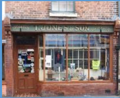
Figure 3 Mid-19th century building and late 19th century shopfront, Leg Street. Henry Thomas.
