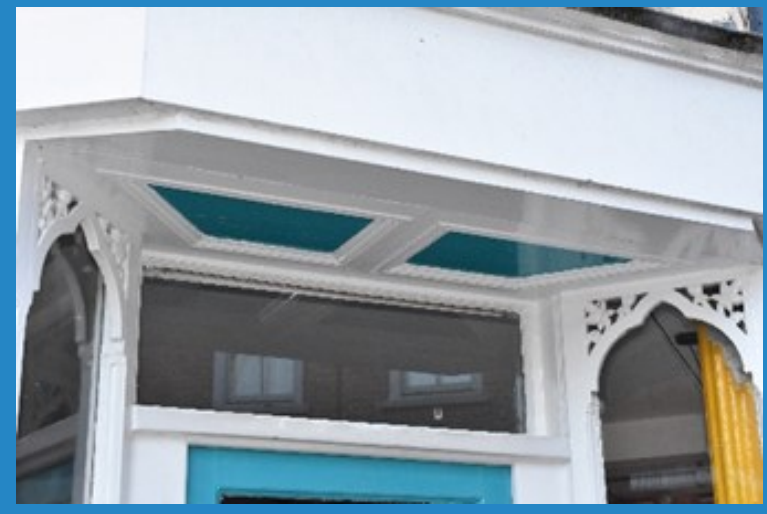
Figure 24 Recessed doorways are part of the character of traditional shopfronts. Details such as door panelling, mouldings and letterboxes can be retained and enhanced, as can tiled or decorative stallrisers.
