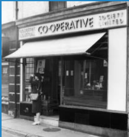
Figure 42 Traditionally retractable blinds were functional and unobtrusive. Cross Street Survey, 1960. Shropshire Archives.
