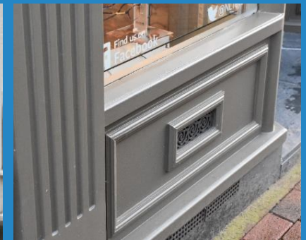
Figure 37 Metal grilles are both practical and decorative. They have been effectively incorporated into this modern shopfront on Church Street.
