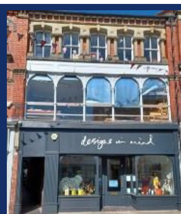
Figure 47 Reinstated shopfront, 2023. Samantha Jones.
