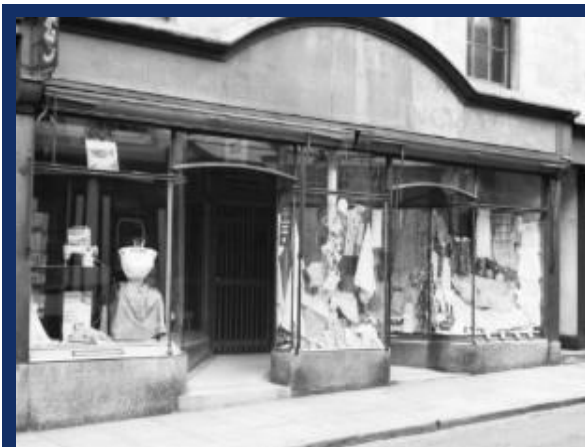
Figure 11 This early 20th century shopfront on Bailey Street spanned the frontage of an early 19 th century building. Cross Survey 1960, Shropshire Archives.
